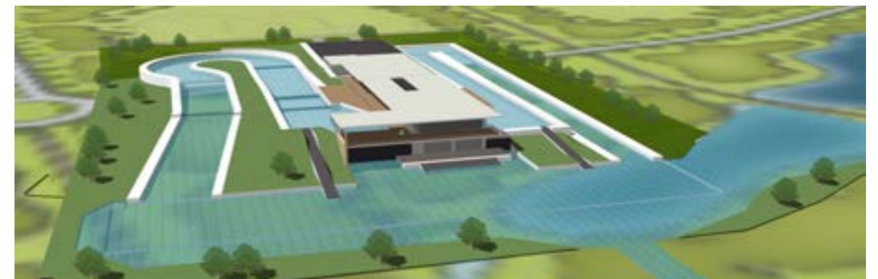
Extract from 3D model - with finishing pond in foreground. Concept shows 2 channels either side of central building
